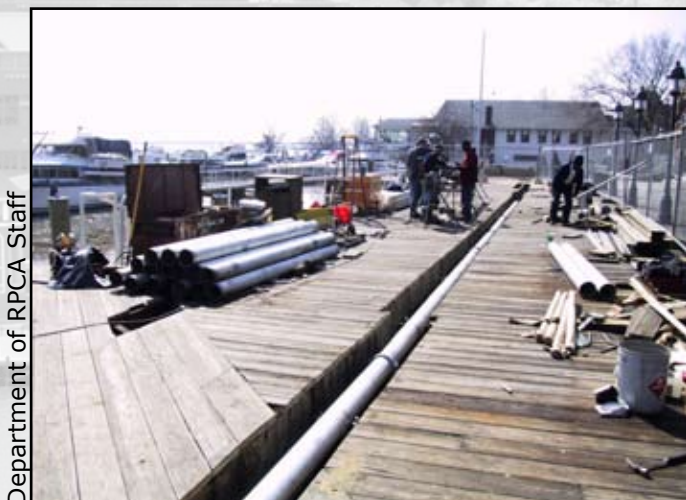
2002 Fire Suppression Project
