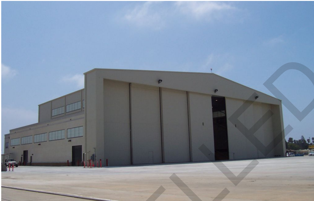
Figure E-5: Large Body Aircraft Hangar with Attached Shops and Office Space and Sliding Doors
