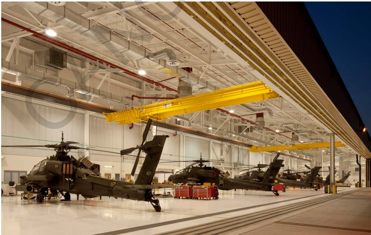
Figure E-6: Helicopter Hangar Bay with Sliding Doors, Sliding Door Tracks and Overhead Cranes
