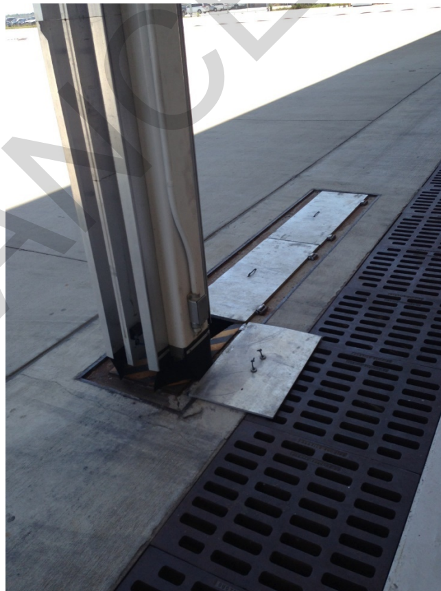
Figure E-14: Vertical Lift Fabric Door Mullion and Mullion Pit
