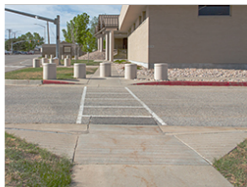
Curb Ramp at Intersection
