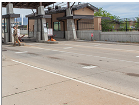
Concrete Paving where Functionally Required
