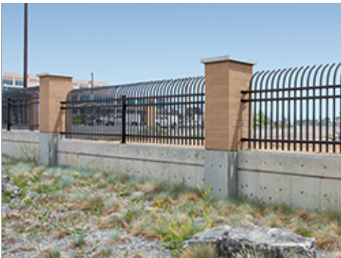
Brick Columns and Metal Fence at Group 1
