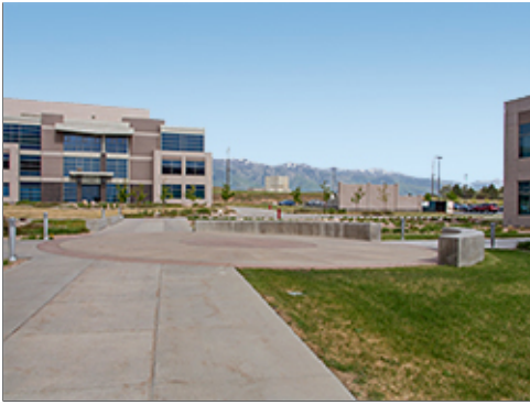
Concrete Plaza at Group 1
