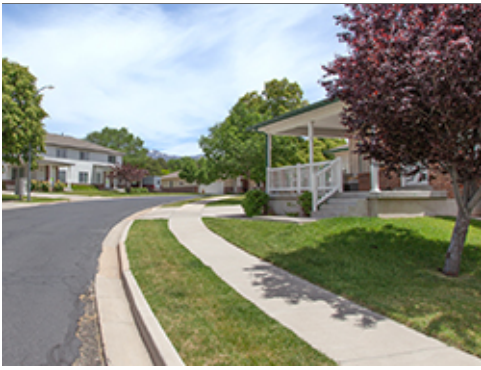
Detached Concrete Sidewalk at Group 4
