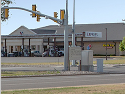
Standard Utility Cabinets
