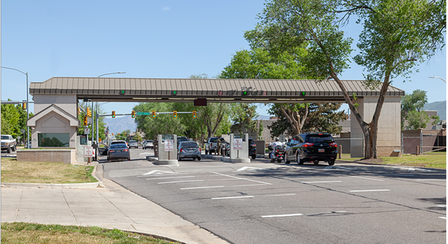
Main Gate at South Gate Avenue
