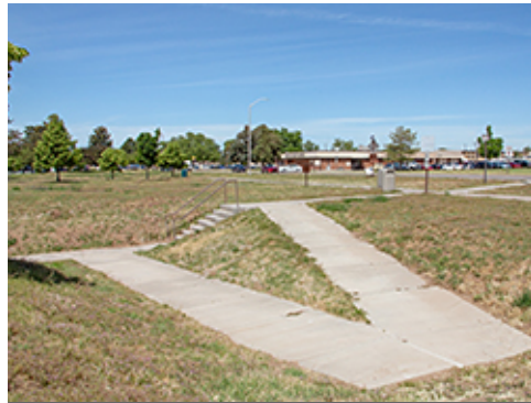
Stair with Integrated Site Ramp
