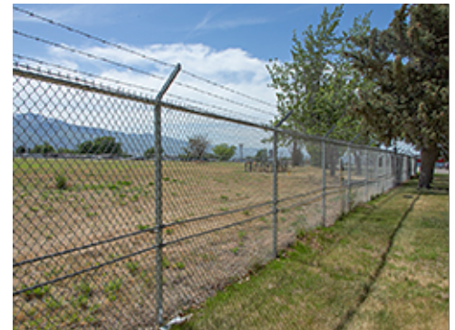
Chain Link with Outriggers at Group 3
