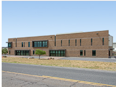
Group 2 Use of Concrete Masonry Units (CMU)
