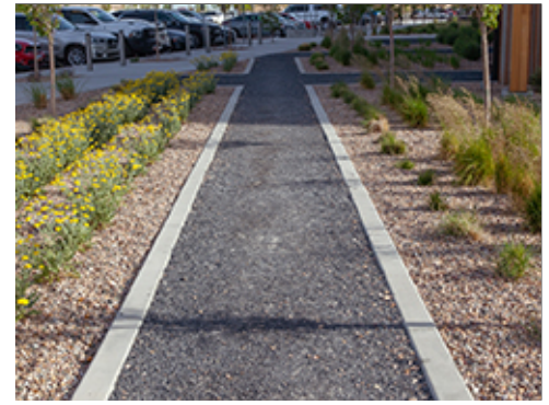
Asphalt Paving in Lansdcaped Area
