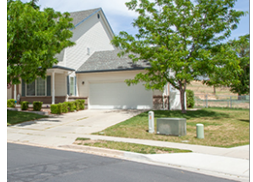
Utility Elements in Group 4
