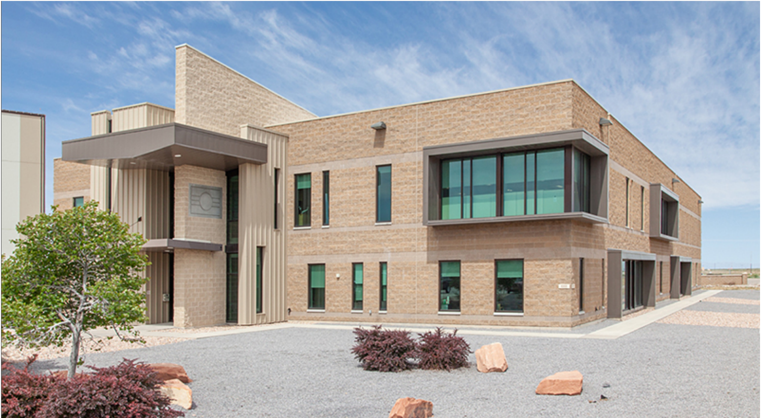
Projections at Windows Providing Shading
