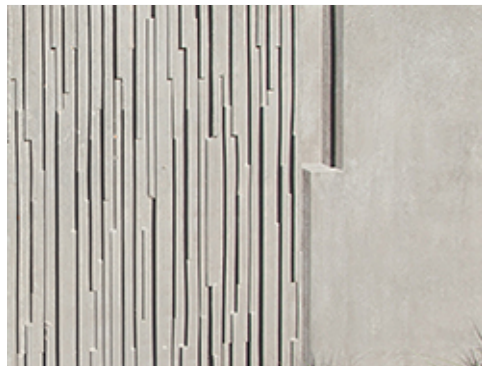
Textured Concrete at Group 1
