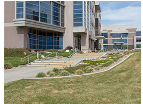
Site Stair at Group 1
