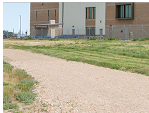
Gravel Paving at Limited Access Area
