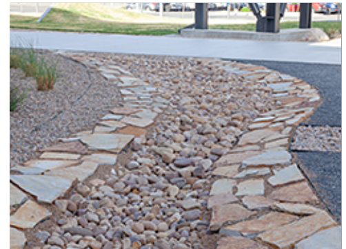
Stone Rip-Rap and River Rock Basin
