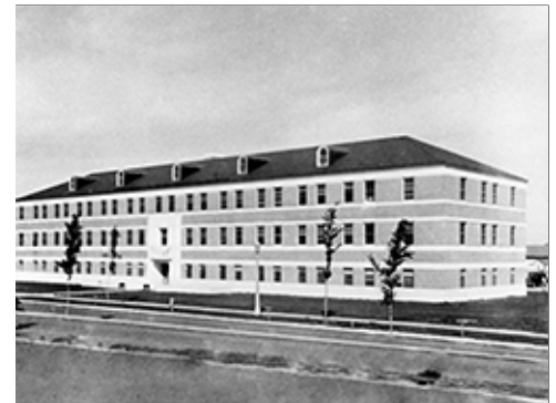
Barracks and Post Exchange, Hill Field, 1941
