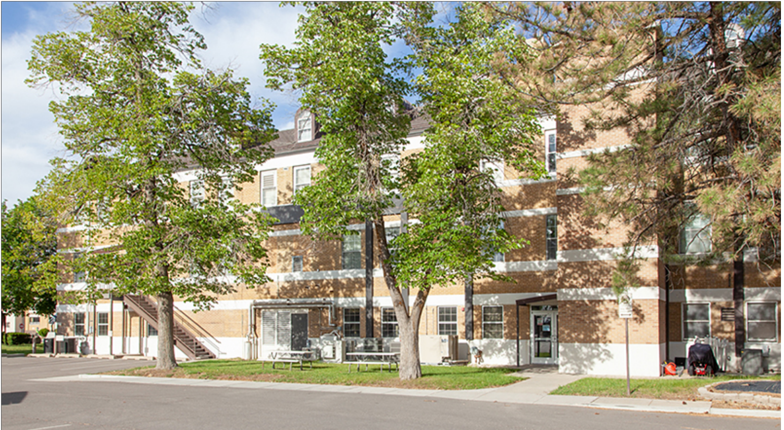
Trees Shading Facade
