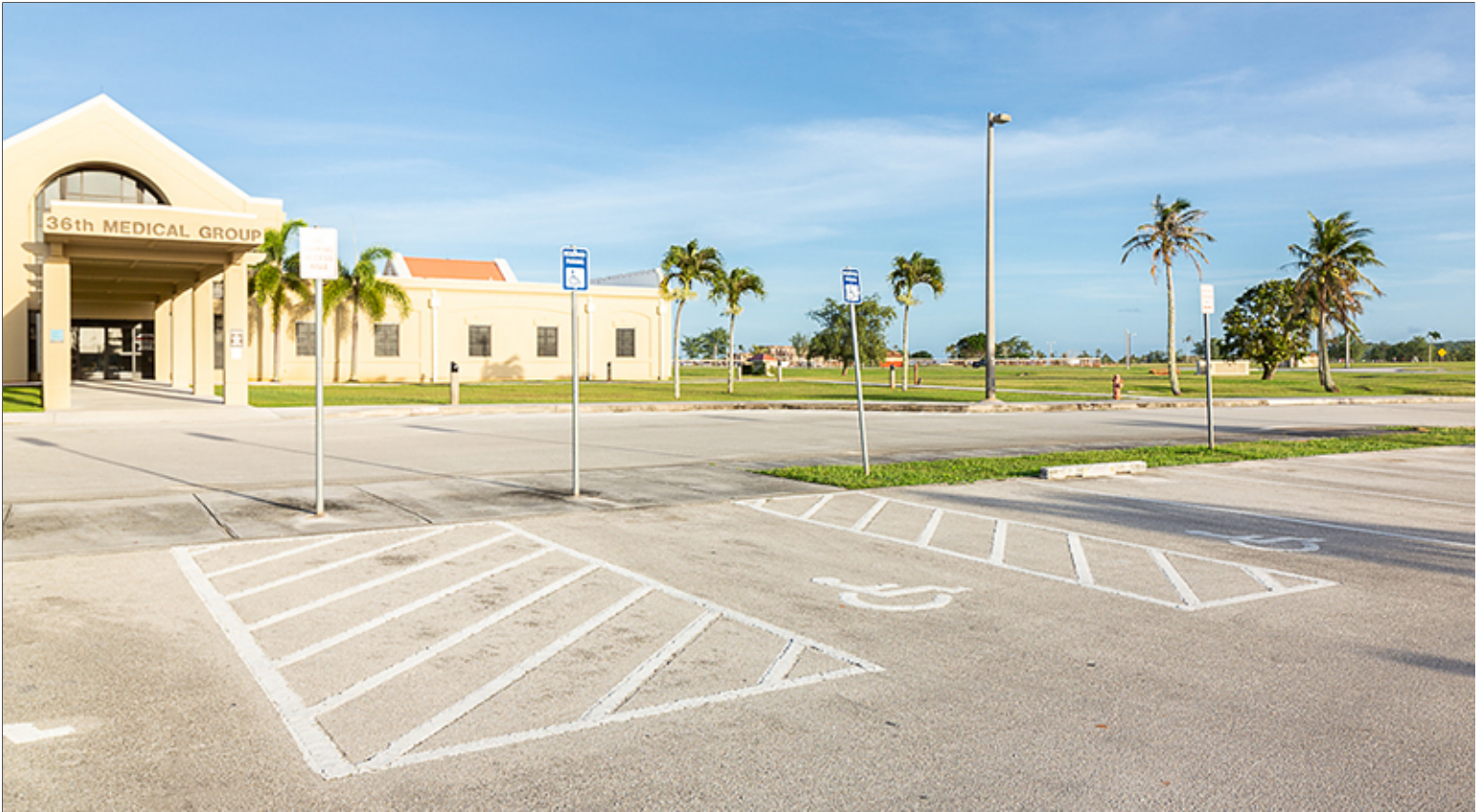
Direct Link to Main and Secondary Entrances
