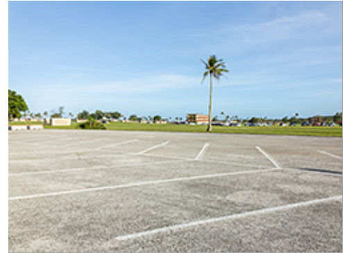
Asphaltic Concrete with White Striping
