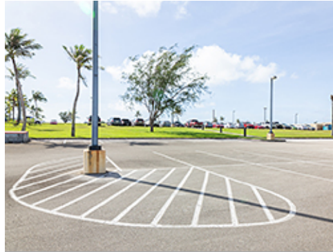
Asphaltic Concrete with White Striping
