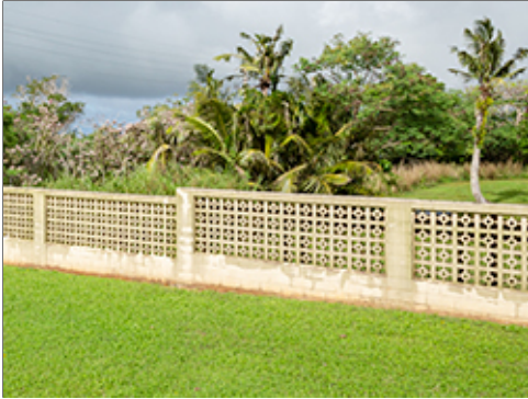
Perimeter Fence at Main Gate
