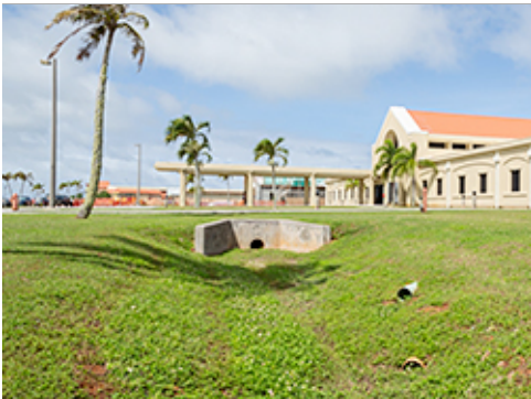
Stormwater Providing Irrigation
