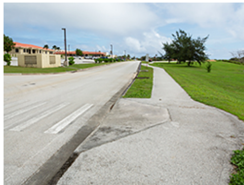
Curb Ramp at Crosswalk
