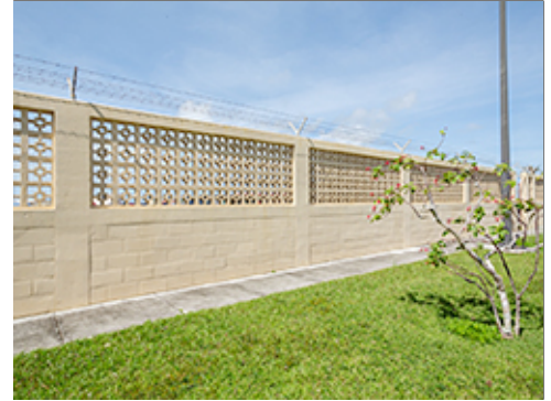
Perimeter Fence at Group 3
