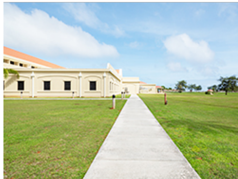
Concrete Sidewalk at Group 1
