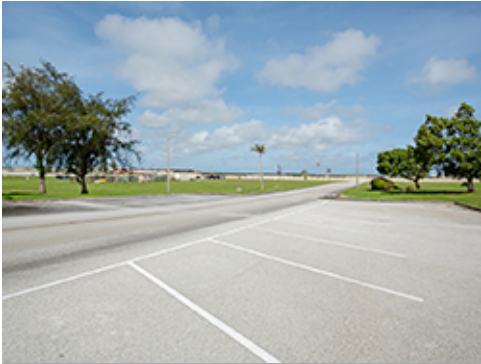
Asphaltic Concrete with White Striping
